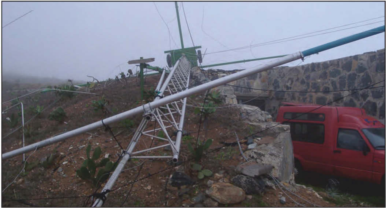
Photo B. Hurricane Delta in 2005 destroyed all six towers and 10 antennas, striking immediately after the conclusion of the CQWW CW Contest.
